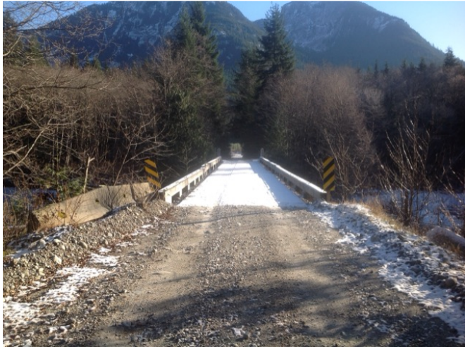
Approach from Right Bank when facing downstream
