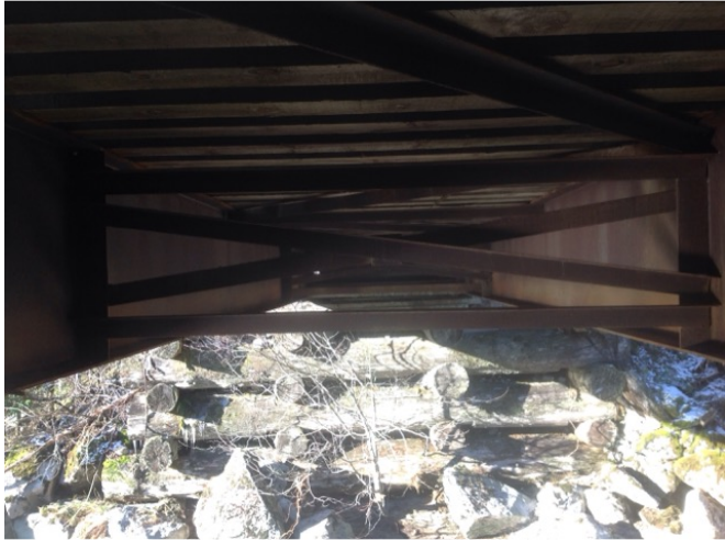
right span superstructure
