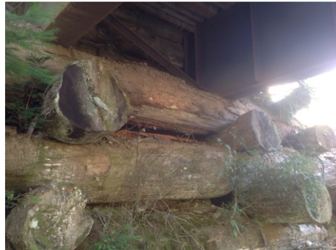
top crib log on left abutment
