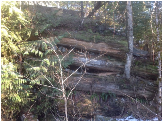
wing wall left approach downstream
