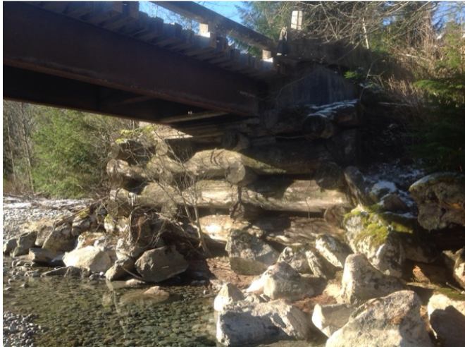
Right Bank Abutment when facing downstream
