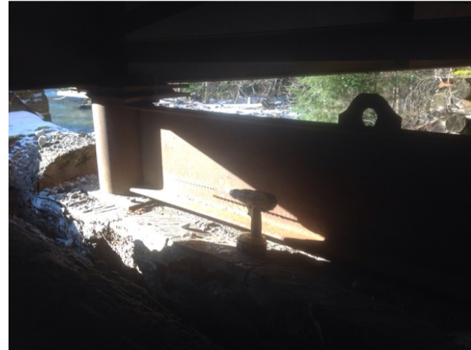
right span pier bearing
