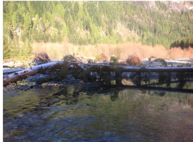
debris at inlet
