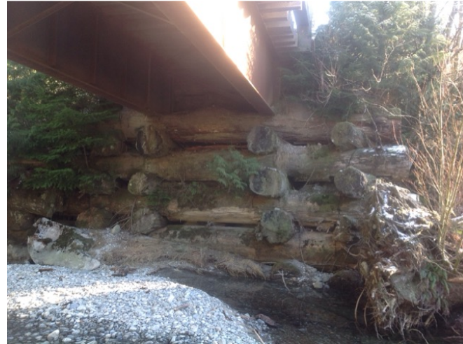
Left Bank Abutment when facing downstream
