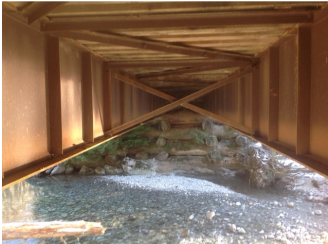
left span superstructure
