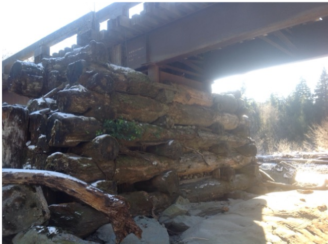
right side of pier
